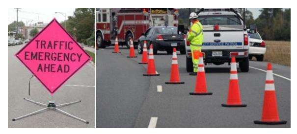
Figure 23. Advance Warning Signs and Traffic Cones (source: mcftoa.org)
